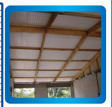
It is recommended a distance of 0 meters to 1.20 meters between supports.
